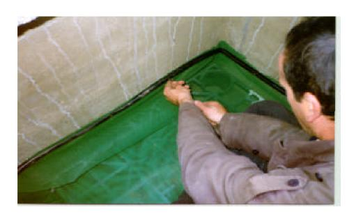
The compost bed consists of 50 mm of coir compost or other coarse fibrous equivalent. This should be spread evenly over the netting to a depth of 50 - 100 mm. (120 -240 litres broken up if compressed)
